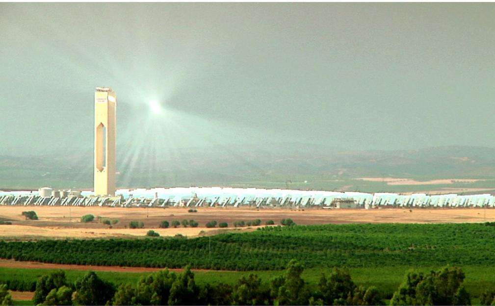
**The Solucar Concentrating Solar Station, outside Sevilla, Spain, focuses the sun's heat on a receiver at the top of the tower.**
